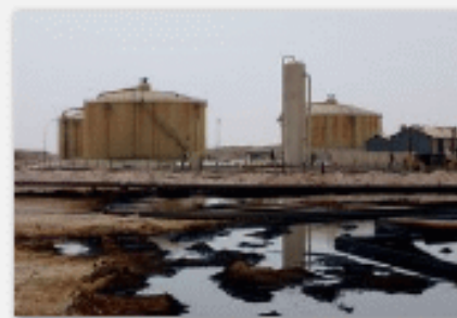
Leakage from petrol storage tanks
